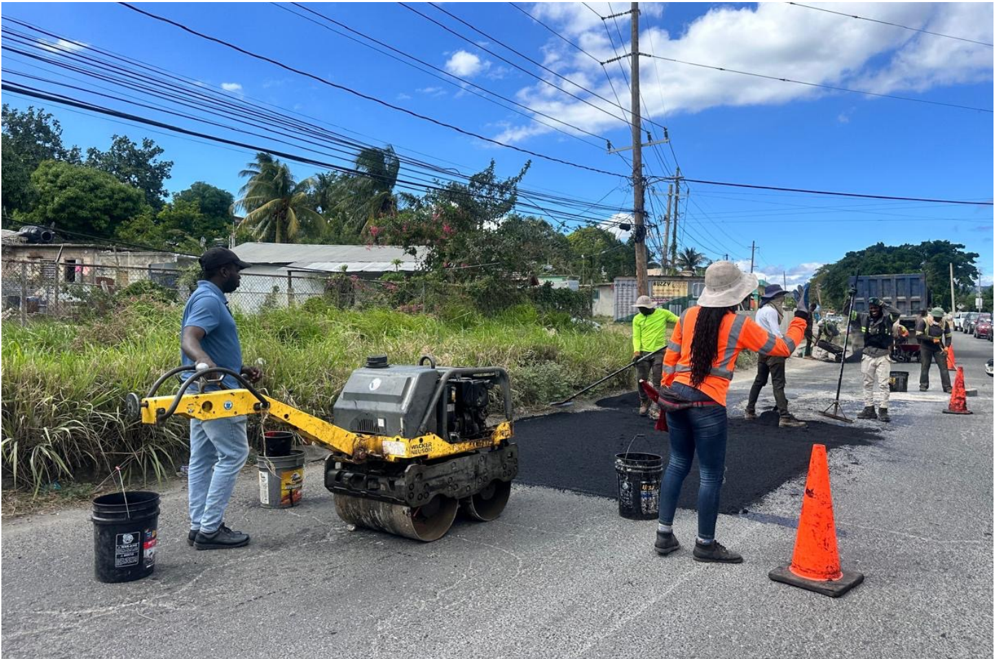
GO ROAD REHABILITATION - ANGELS CRESCENT, ST. CATHERINE
