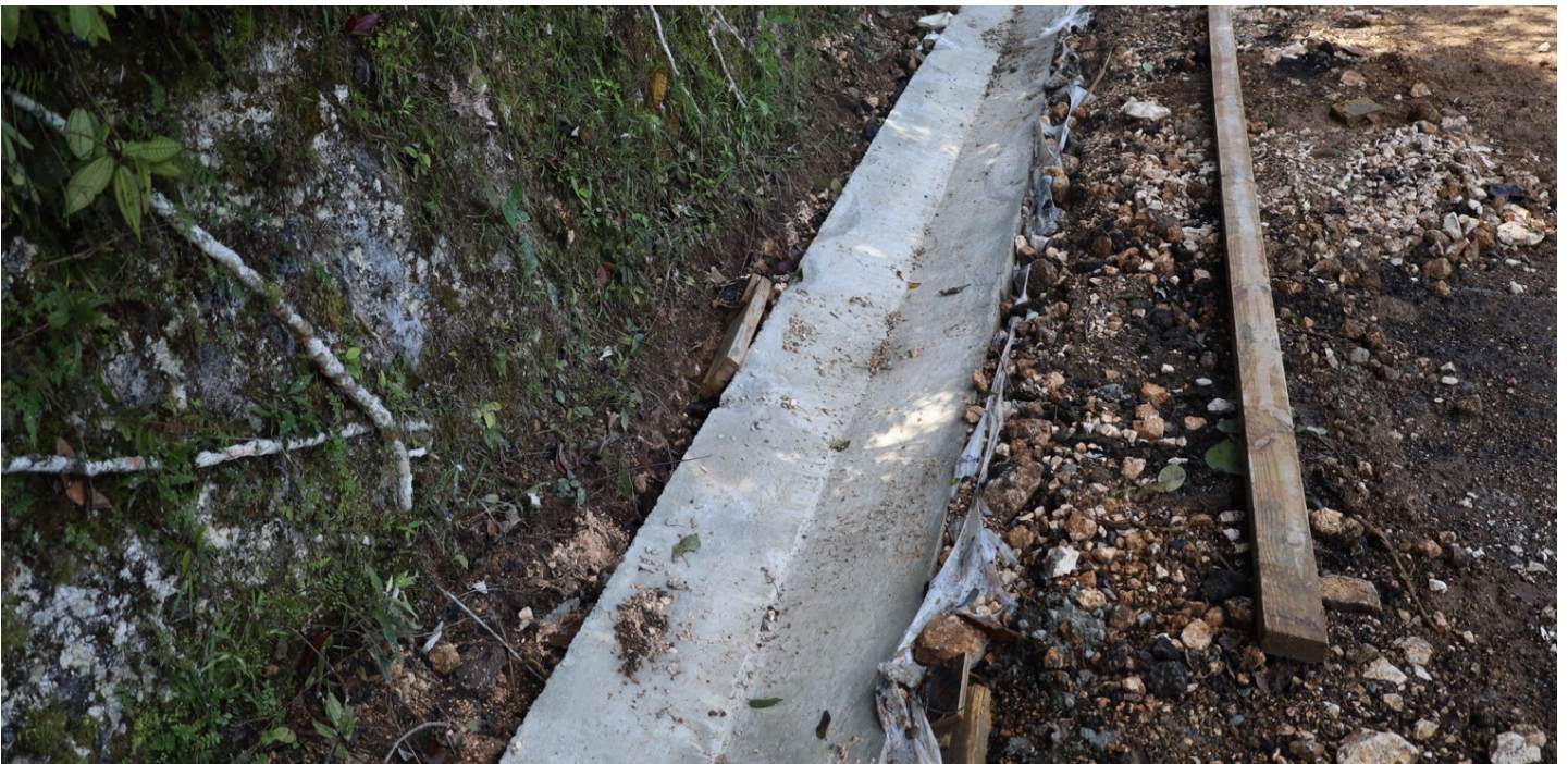
GREENDALE CRESCENT, ST. ANDREW - COMPLETED V DRAIN FORMATION ON SPARK ROAD
