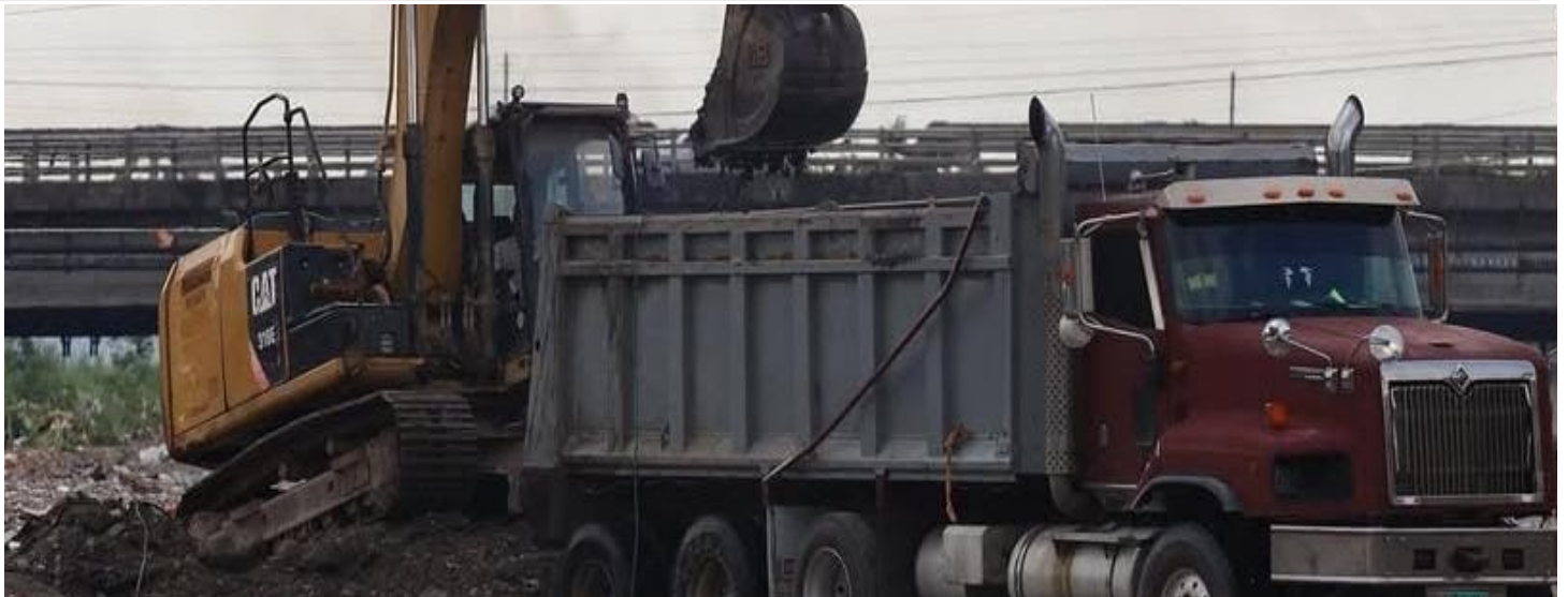
GULLY MAINTENANCE - SANDY GULLY - ST. ANDREW WESTERN
