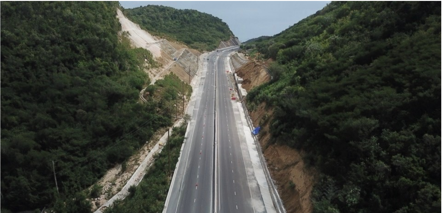
AERIAL VIEW OF SOUTH-COAST HIGHWAY IMPROVEMENT PROJECT (SCHIP)
