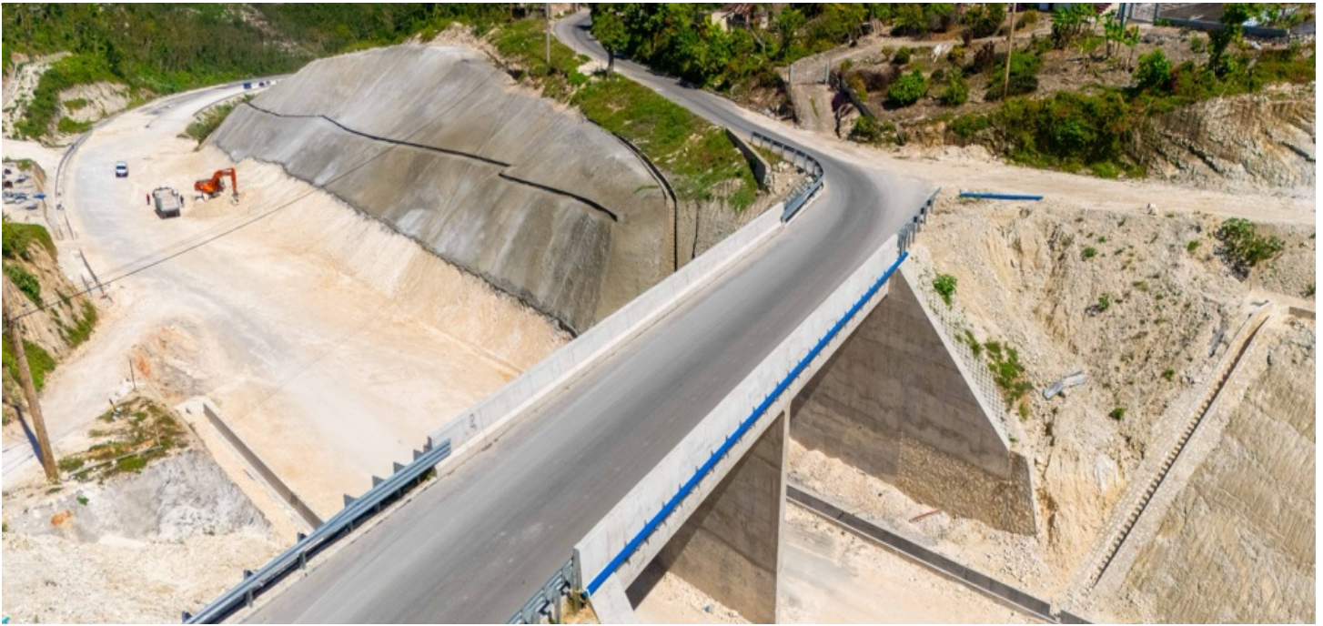
MONTEGO BAY PERIMETER ROAD - COMPLETED ASPHALT WORKS AS AT MAY 21, 2026
