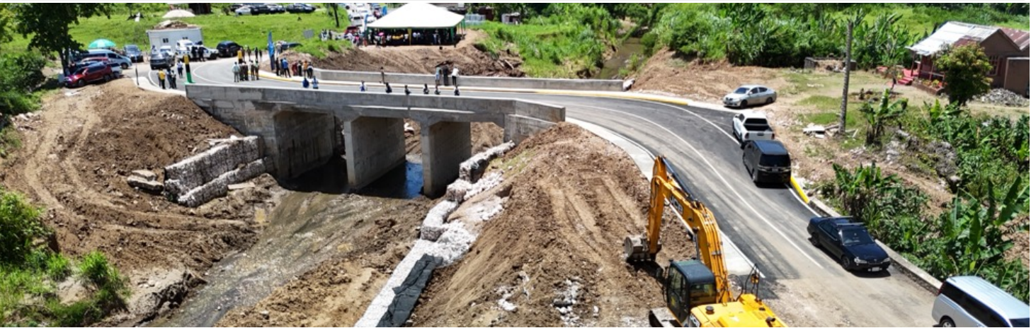
AERIAL VIEW OF TROY BRIDGE
