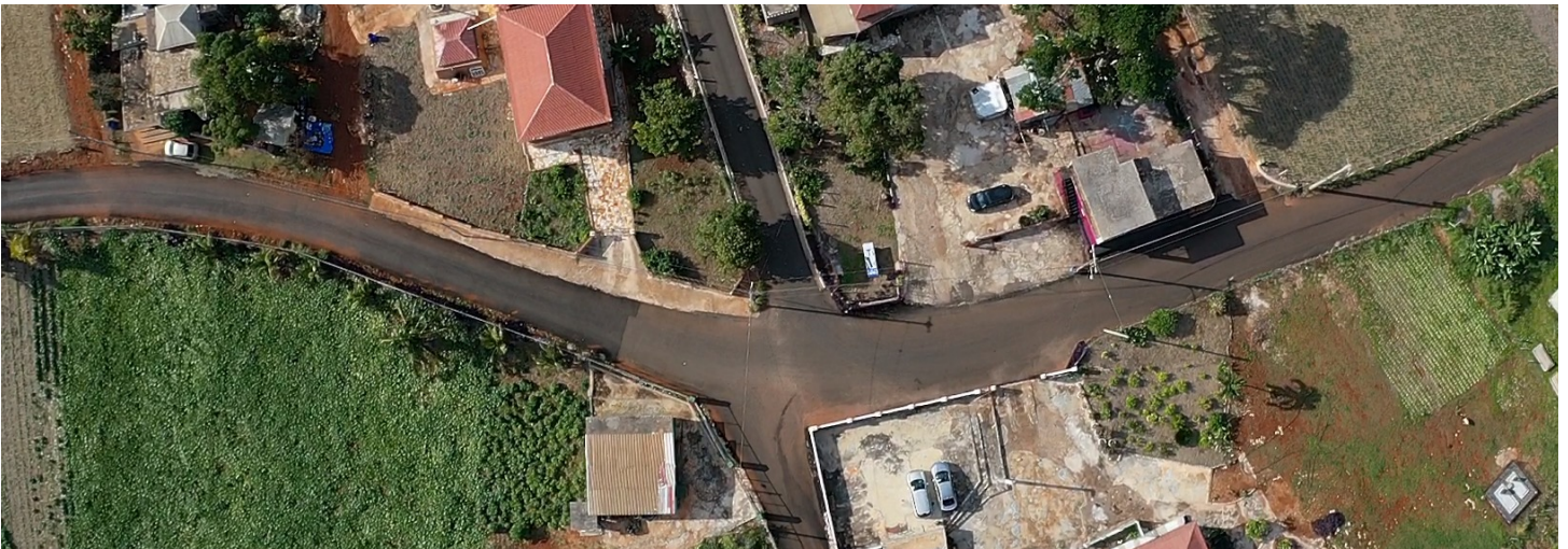
SPARK ROAD- BARNSTAPLE, MANCHESTER - COMPLETED
