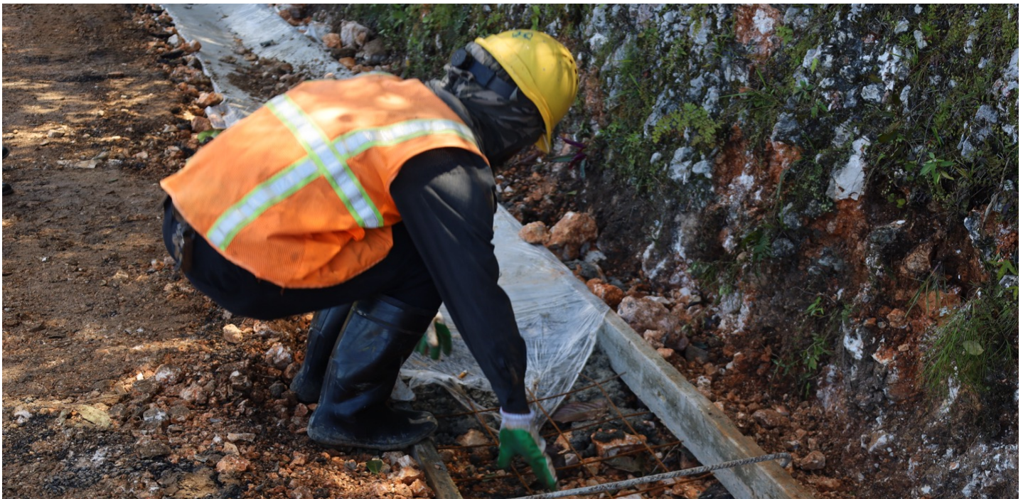
GREENDALE CRESCENT, ST. ANDREW - V DRAIN FORMATION ON SPARK ROAD
