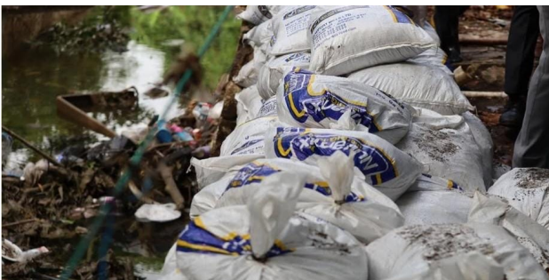
GULLY MAINTENANCE - BURGHER GULLY - EAST KINGSTON
