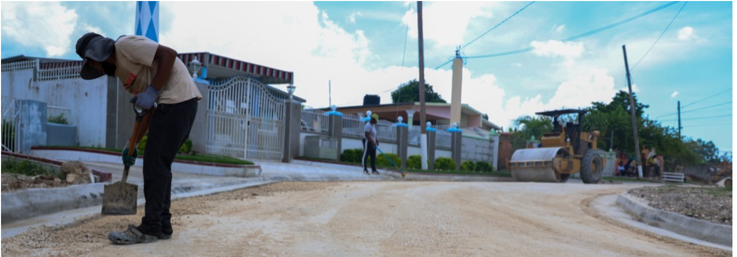
SPARK ROAD GREENDALE CRESCENT, ST. ANDREW (NOW COMPLETED)
