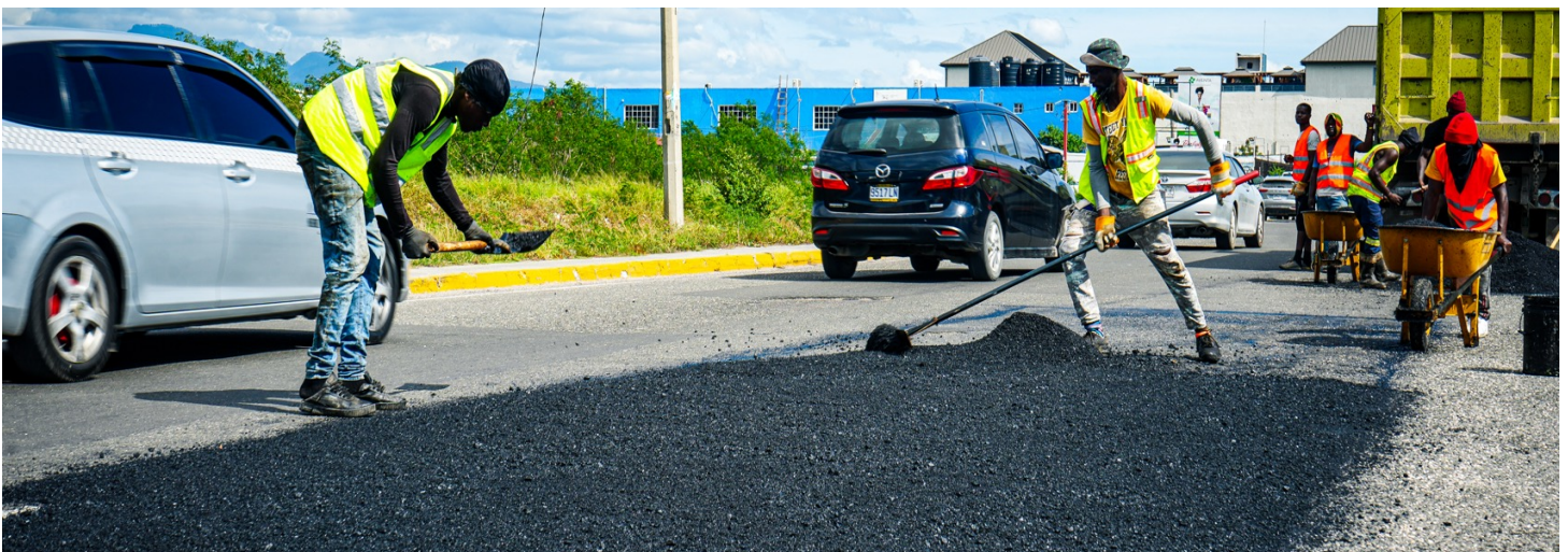
ROAD MAINTENANCE - PORTMORE
